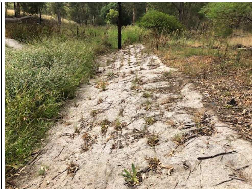
Photo 2 – BC4 - March 2019 – Planted jute matting – southern bank with insufficient density and poor growth – contingency planting required
