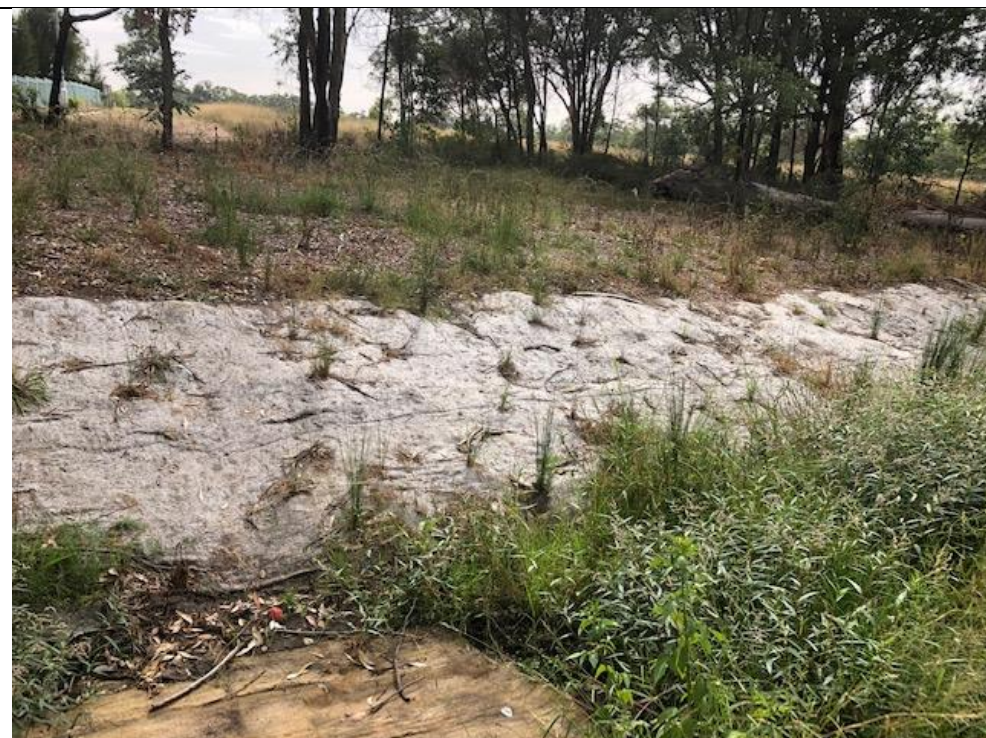
Photo 2 – BC4 - March 2019 – Planted jute matting –northern bank with insufficient density and poor growth – contingency planting required
