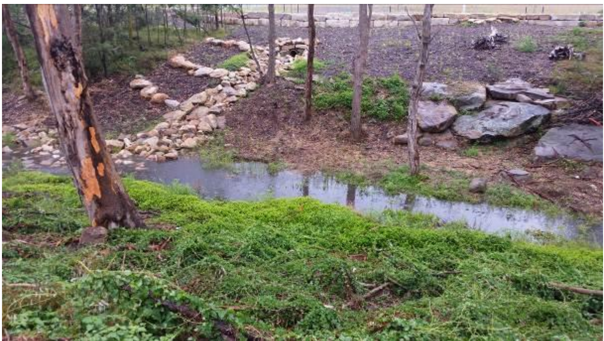
Photo 12 – Looking from the same Madeira Vine area of Photo 11, across the creek to the stabilised stormwater outlet in Photo 6
