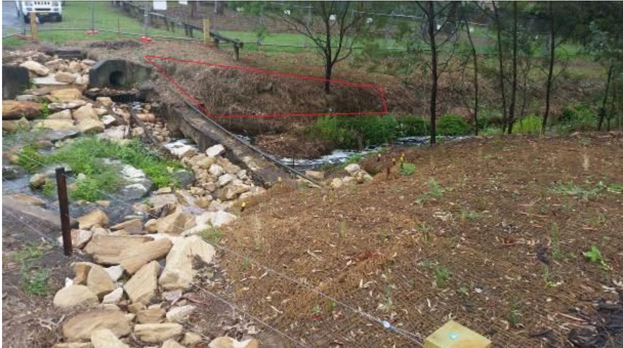
Photo 1 – Minor erosion occurring on north side of College Road on the western side of creek (red polygon). The eastern side of the creek is stable with jute mesh and planted tubestock
