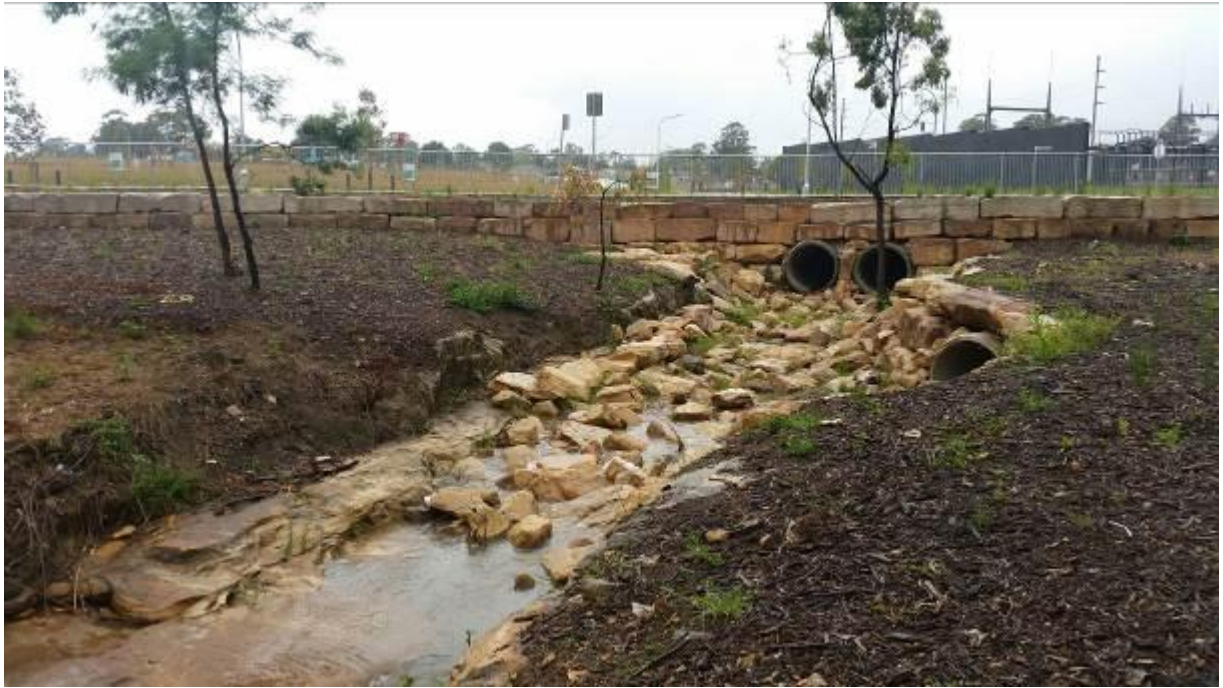
Photo 5 – Stabilised stormwater outlets off the eastern boundary closer to College Road
