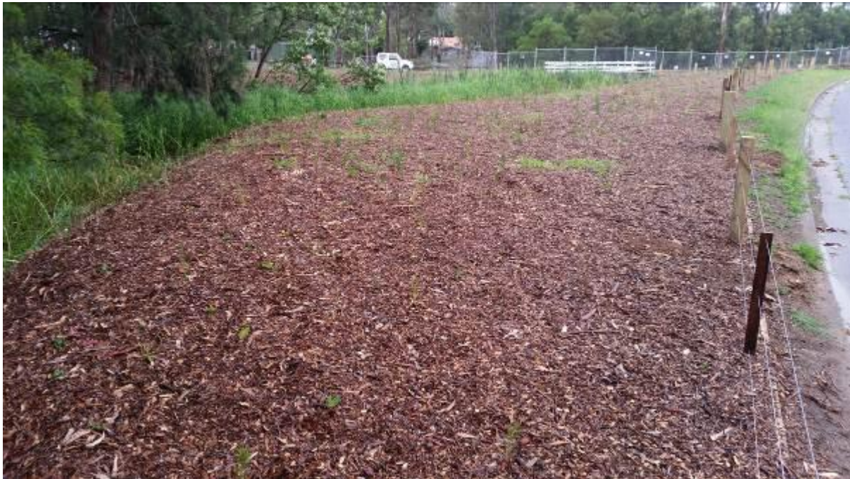
Photo 14 – Newly revegetated and mulched southern portion of BC1
