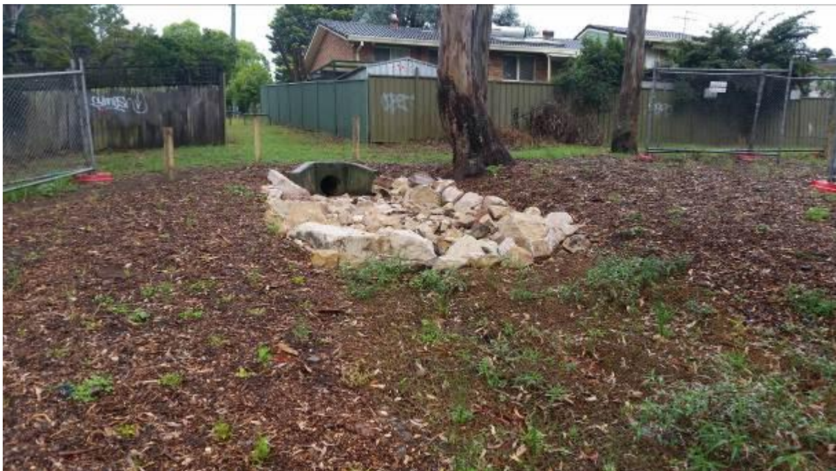
Photo 4 – Stabilised outlet on western side of creek, between College Road and Georges River Road
