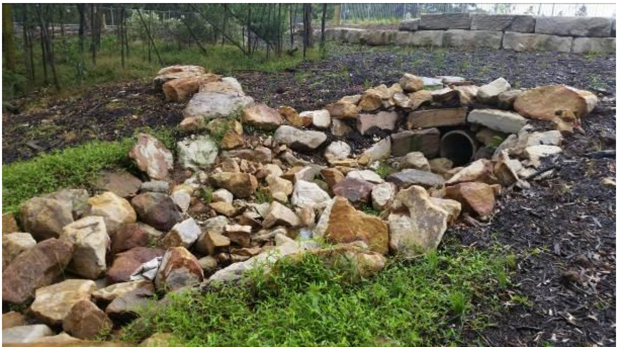
Photo 6 – Stabilised stormwater outlets off the eastern boundary closer to Georges River Road
