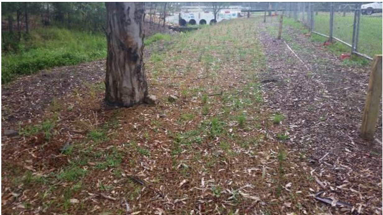
Photo 2 – Partially jute matted embankment. Planted with grasses, tussocky species and occasional shrubs. Planting density varies between 4 and 8 plants per m 2 .
